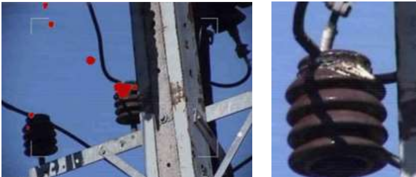
Fig. 9, 10. Corona discharge and its effects.
